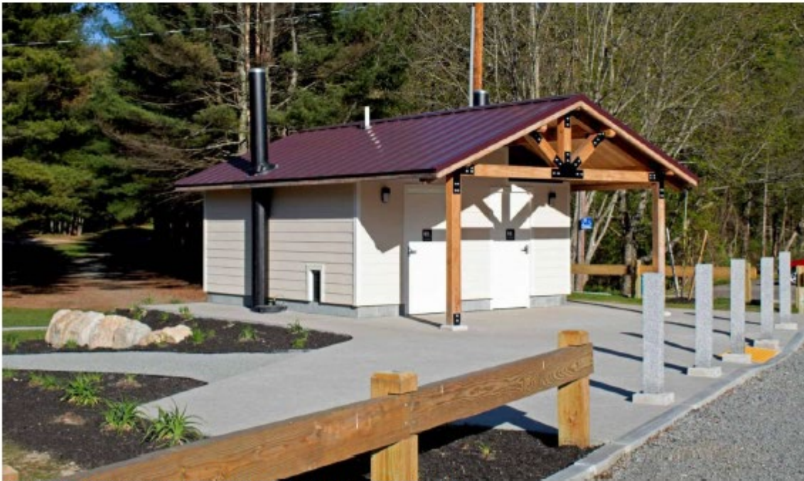
Figure 4 - Modern-style Block Prefabricated Restroom Building
