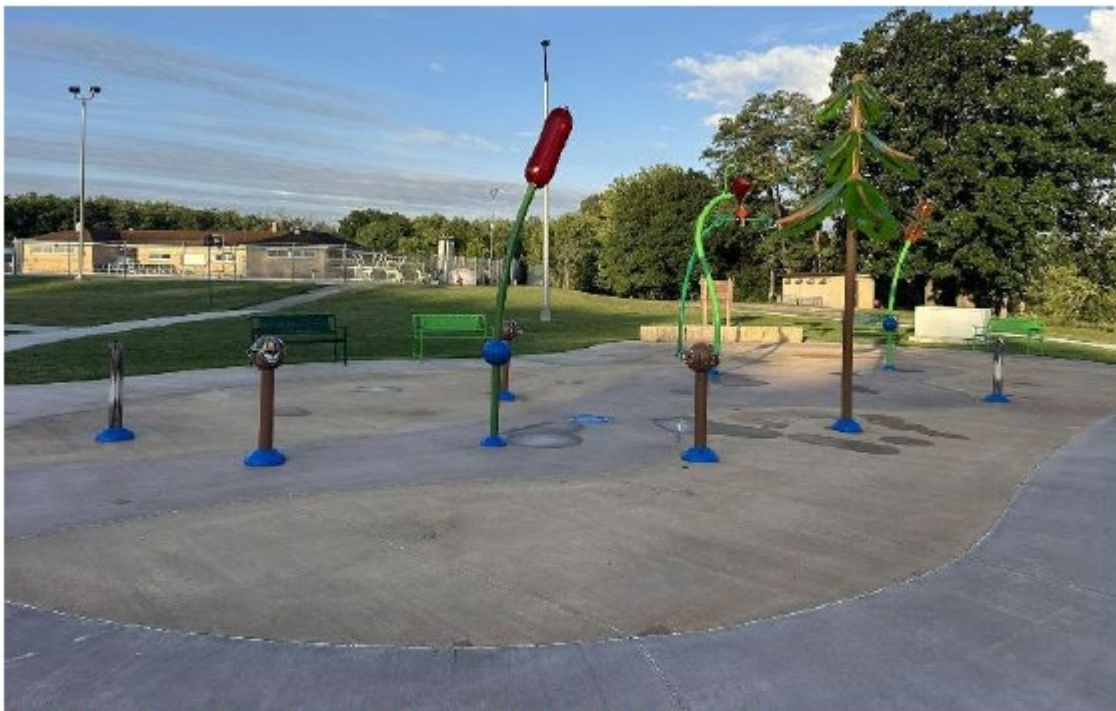
Figure 5 – Site photo of splashpad install at Legends Park in Reedsburg WI
