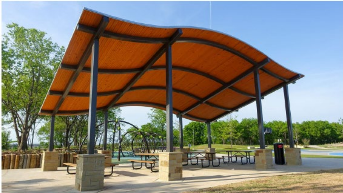
Figure 2 - Alternate Metal Canopy Structure (25' x 40')
