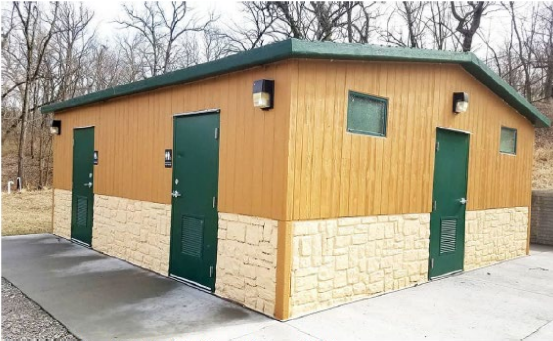
Figure 3 – Traditional-style Block Prefabricated Restroom Building
