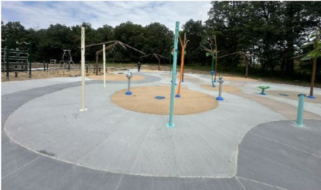
Figure 8 - Site photo of splashpad install at Legends Park in Reedsburg WI
